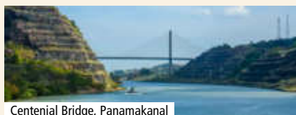
Centennial Bridge, Panamakanal
